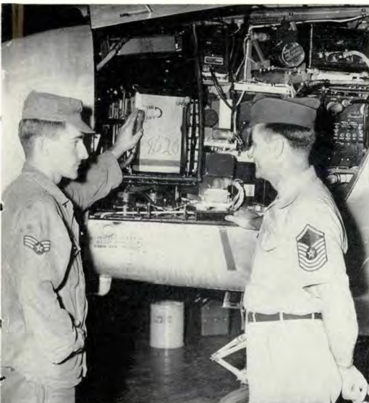
Q. Which way are the battery connector fiber nuts turned to loosen? A. Clockwise. (AIC Joseph Parnell quizzed by SMSgt Benjamin Cliff.)
